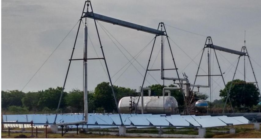
Figure 4.16: An LFR system installed at Vallipuram, India; Reprinted from Chaitanya Prasad, Reddy, and Sundararajan (2017), Copyright (2017), with permission from Elsevier
