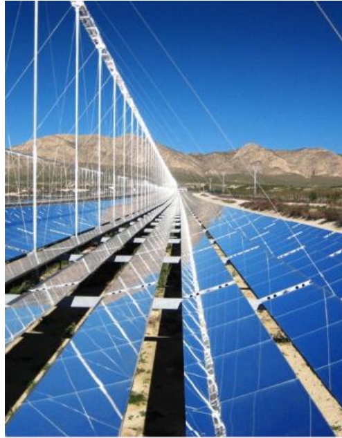
Figure 1.6: Puerto Errado 2, a 30MW LFR power plant located in Murcia, Spain (Zhu et al. 2014), Copyright (2014), with permission from Elsevier
