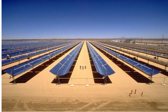
Figure 1.3: A 30MW parabolic trough power plant located at Kramer Junction in the Mojave Desert, California, USA (U.S. Department of Energy 2003)
