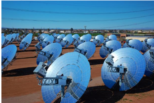
Figure 1.4: The Maricopa solar plant, 1.5MW parabolic dish system, in Arizona, USA (United Sun Systems International Ltd, 2012), licensed under CC BY-SA 4.0
