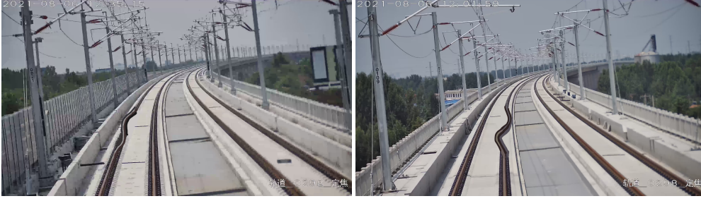
Figure 4.9: Examples of digitally modified images of rail tracks with sun kinks.
